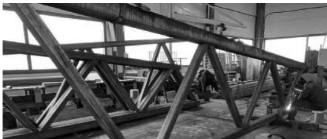
Figure-2. Surface treatment of metal structures
