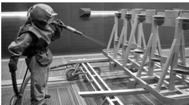
Figure-4. Protection of metal structure from corrosion
